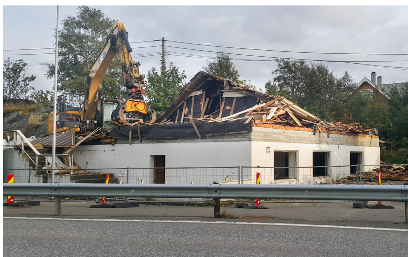
Blom bedehus under riving.
